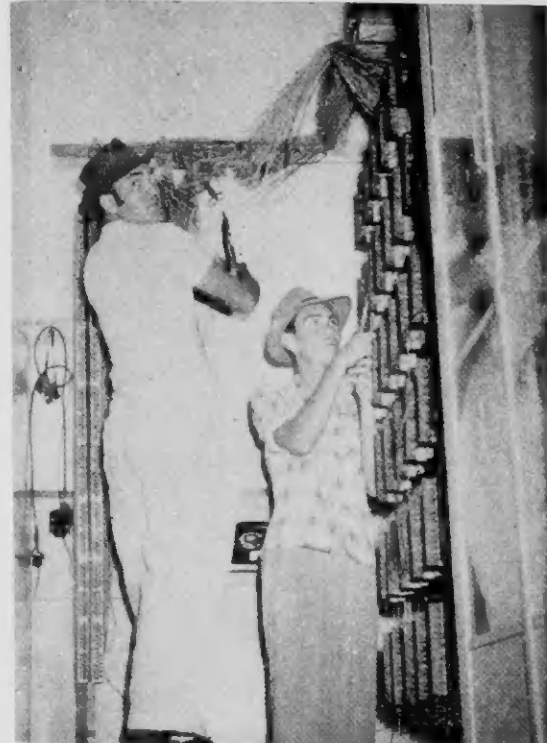
Adolph Arends cuts hundreds of temporary jumper wires that kept the two exchanges linked, while Carlino Henriquez cuts hundreds of old exchange incoming wires.
